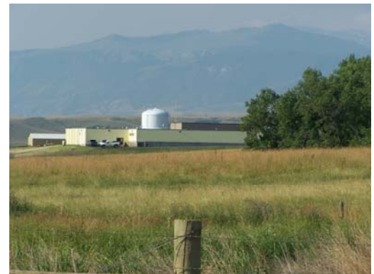
Sheridan Water Treatment Plant
